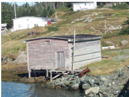
Torraville Stage (Before Restoration)
